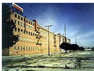
Former Manufacturing Plants
